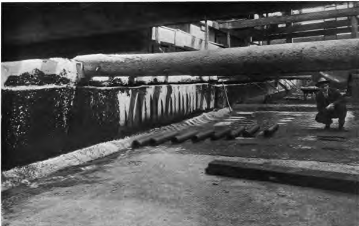
LAYING SHEET WATERPROOFING IN BOTTOM
